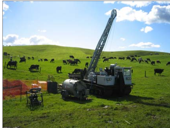
Setting up the drilling rig for the 2 nd hole at Tahunaatara →
